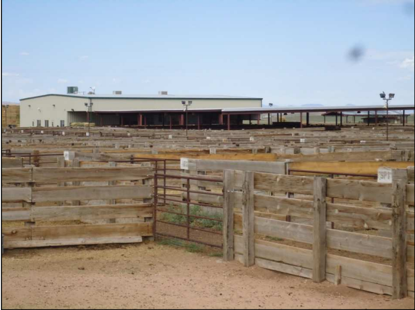
View over the pens toward the backside of the sale barn.
